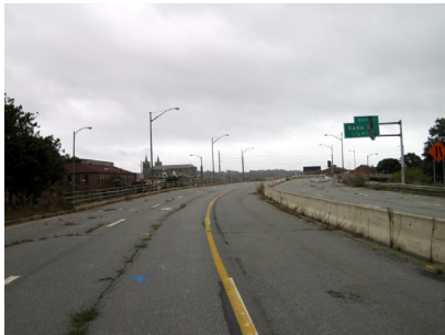
The I-195 Bridge, pre-demolition 4
