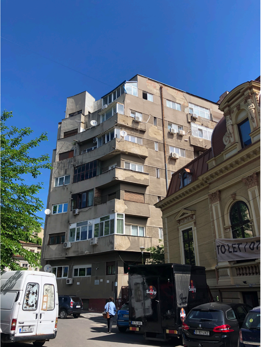
A modern building from the 1920s, photographed in 2019 by the author.
