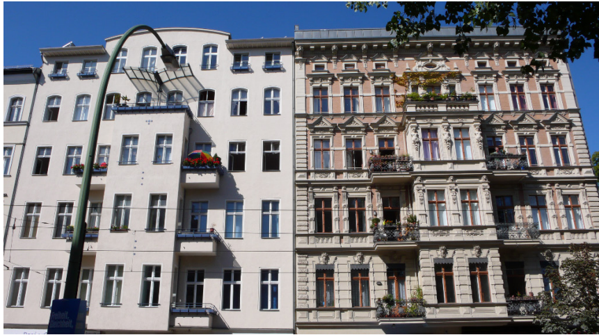
Figure 4. Stucco Facades, Example of Weimar Entstickung, Prenzlauer Berg, Germany, 2009.
