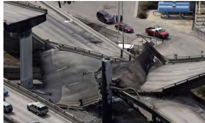
Figure 1.17: The collapse of Atlanta's I-85 interstate in 2007. Source: CNN
