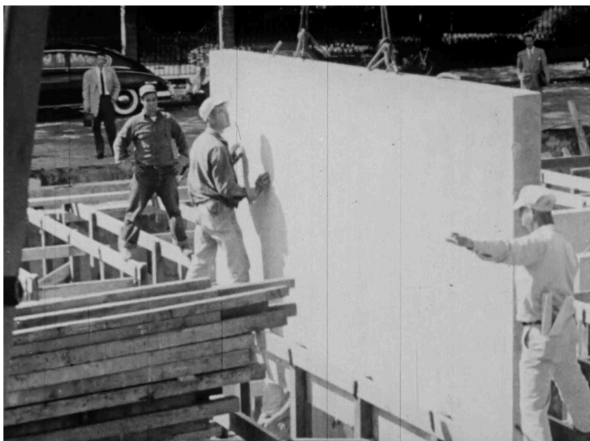
Figure 3. Still from The Quadrangle Story showing construction.
