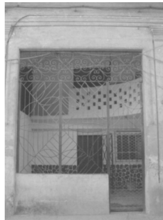
Figure 5 Example of a barbacoa , a two-story contemporary construction subdividing an older colonial structure, meant to increase living space. 43
