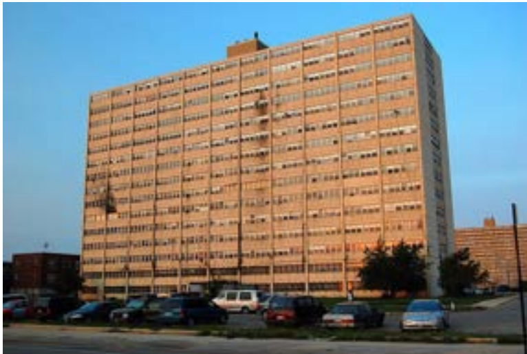
Figure 6 Cabrini Green Housing Complex, Green Towers (Arch.: Charles Genther), 1960, demolished 2010.
