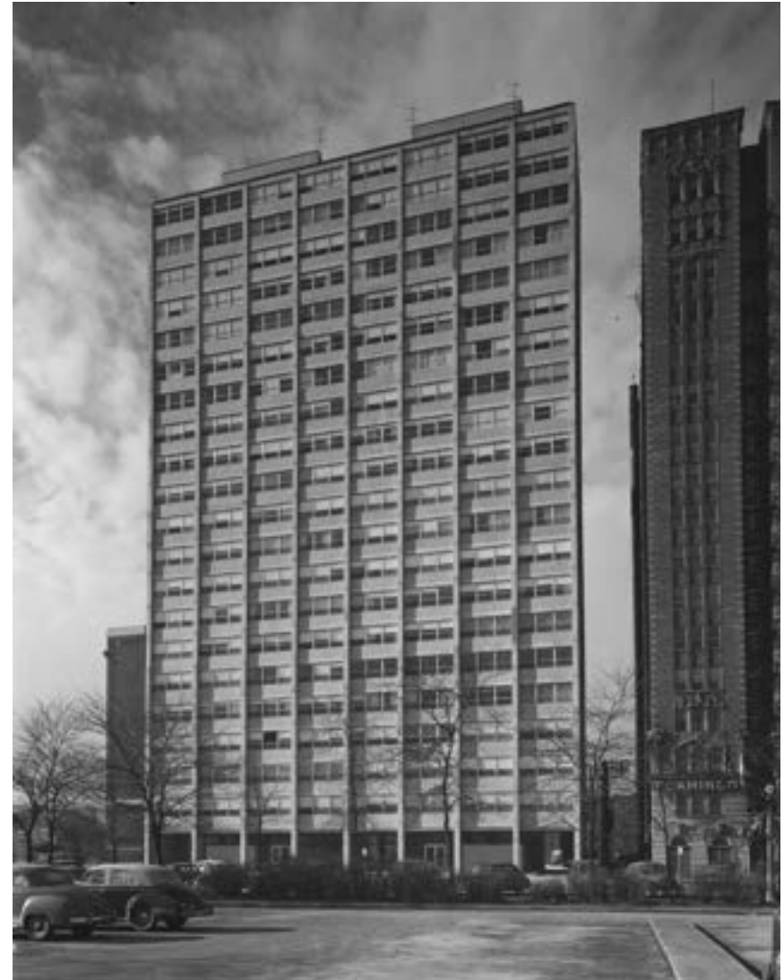
Figure 3 Promontory Apartments, Chicago. Photo: Hedrich Blessing, Chicago History Museum
