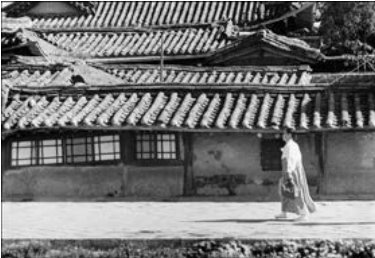
HANOKS ON THE VERGE OF COLLAPSE. PHOTO COURTESY OF SEGYE NEWS .
