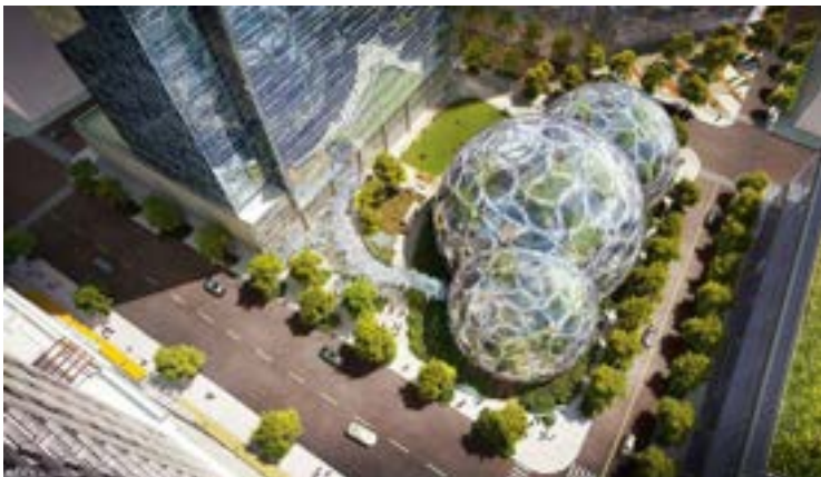
COMPLETED AMAZON SPHERES AT THE DAY 1 BUILDING. PHOTO BY NBBJ DESIGN.
